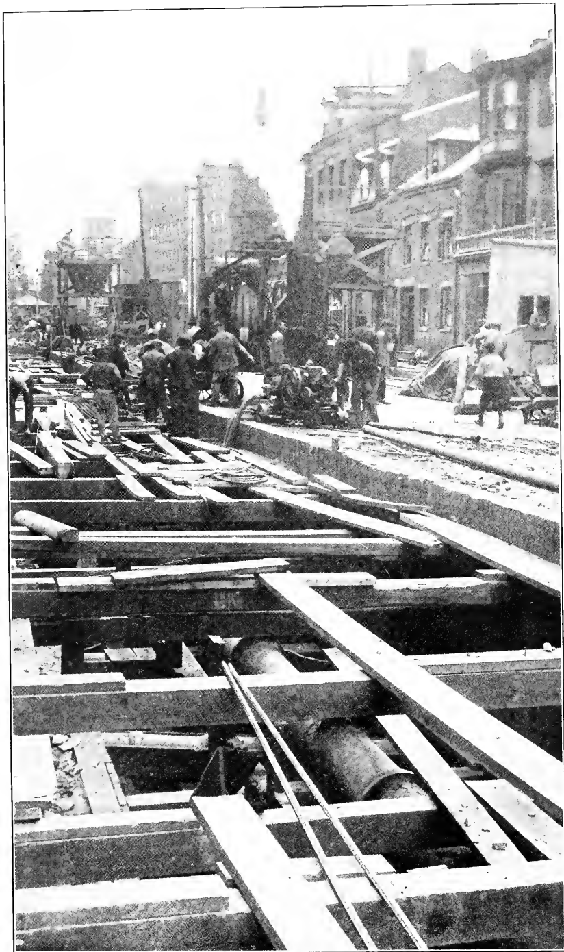
PLATE 2.—TRENCH FOR EAST WALL OF SUBWAY — CHELSEA STREET
